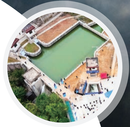
Xiaolangdi South Bank Irrigation Area
