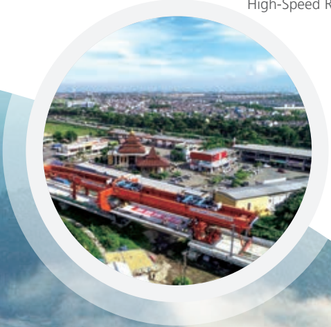
No.4 Beam Field, Jakarta-Bandung High-Speed Railway
